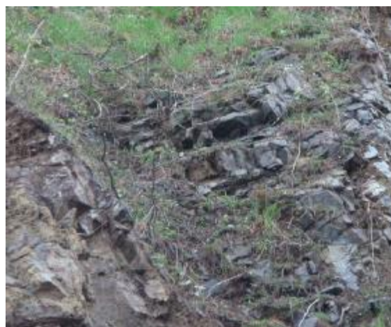
Slika 14. Postojeće stanje – ispucala stenska masa Figure 14. Present condition – cracked slope
