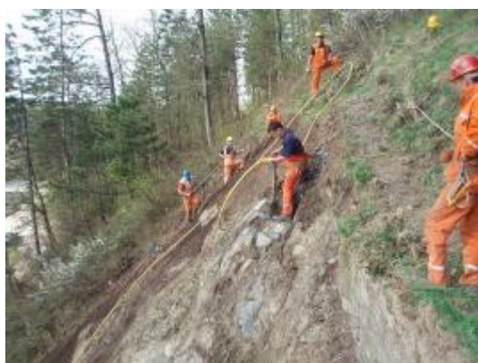
Slika 4. Čišćenje niskog i visokog rastinja Figure 4. Cleaning of low and high vegetation
