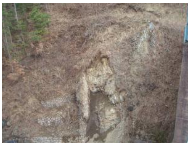
Slika 13. Postojeće stanje Figure 13. Present condition (state)
